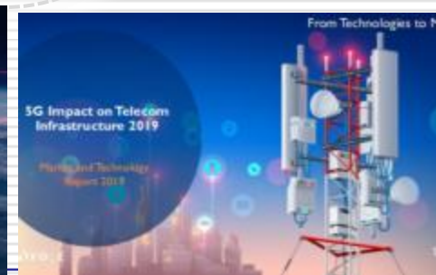
5G Base Station
